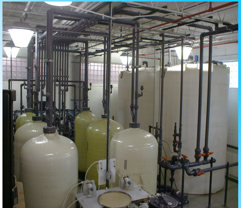
Carbon Filtration and ion-exchange rinse water treatment and recycling system for a plating facility
