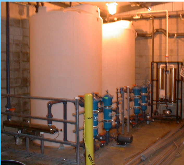
Ozone(O 3 ) treatment system for processing oily wastewater to reduce BOD and COD levels for discharge to POTW
