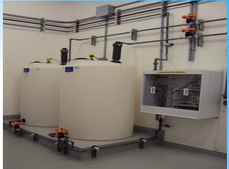
RO and DI water storage and piping systems for manufacture of dairy products
