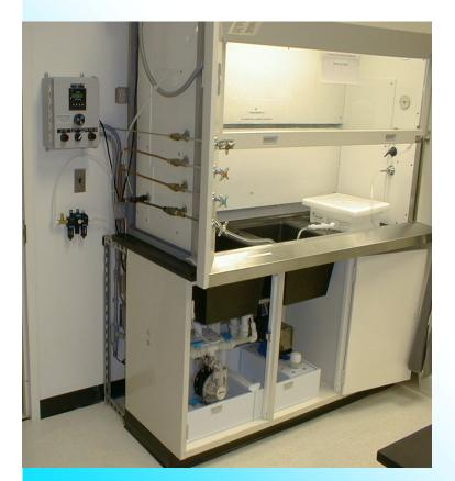
The photo shown to the left is an automated wastewater neutralization system that fits under the sinks in a R&D lab hood.
