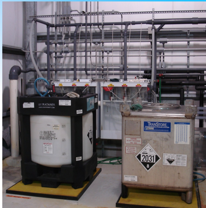
Automated delivery system for hydrofluoric (HF) acid and nitric (HNO 3 ) acid. PLC controlled operation that transfers the acids to three different process tanks through double contained piping.
