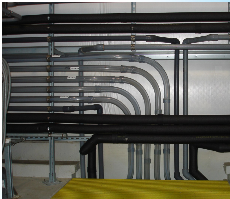
View of chemical and process piping installation, piping systems include acid feed piping (PFA in clear PVC containment), caustic feed piping, waste acid transfer piping, chilled water piping, and process air piping.
