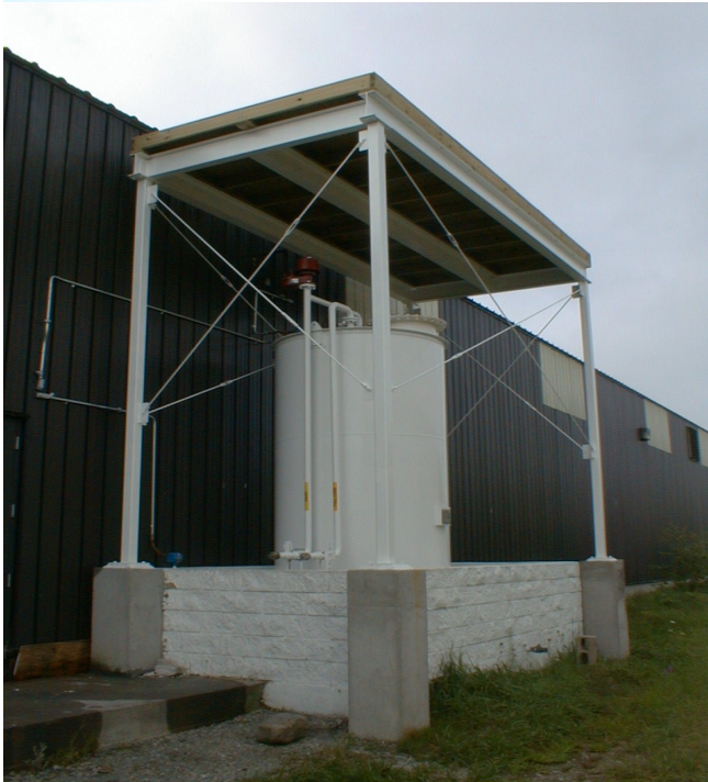
Toluene bulk storage facility showing tank, conservation vent, piping, and containment with roof
