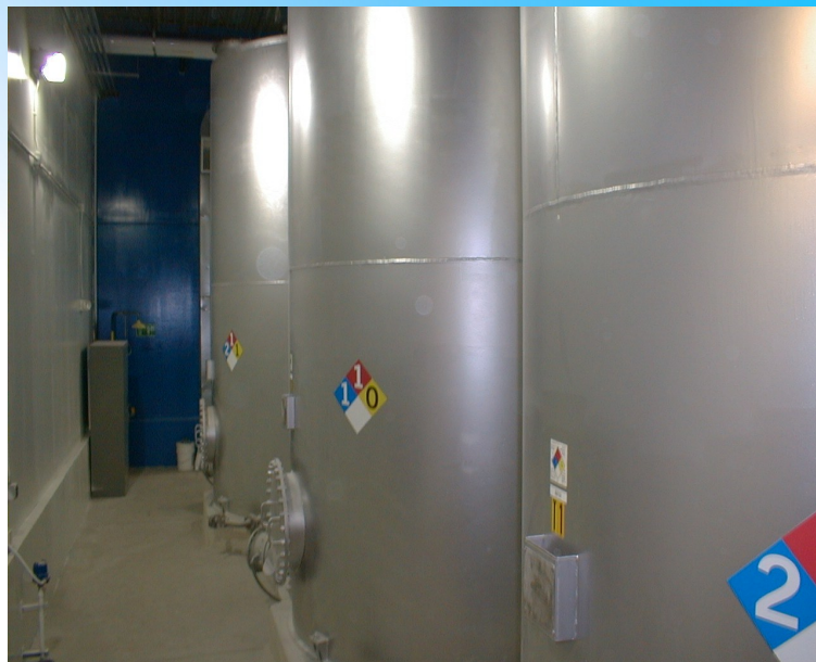
Resin bulk storage facility with painted carbon steel tanks. PLC automated piping system that controls the temperature and delivery of the resins to production.
