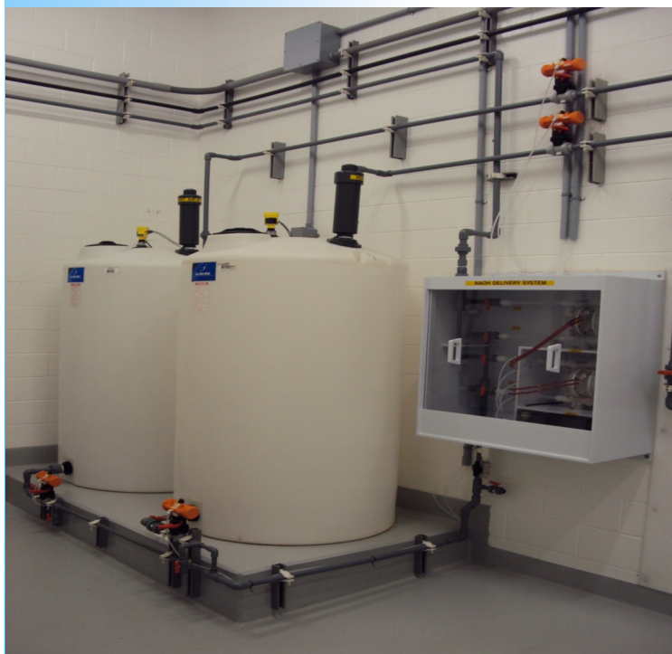
Sodium hydroxide storage and delivery system with inline mixing capabilities. The system automatically dilutes and delivers NaOH solution to production.
